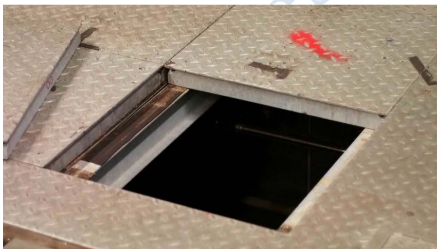
Figure 4-10. Manholes utilized for inspection of the underground volume.
