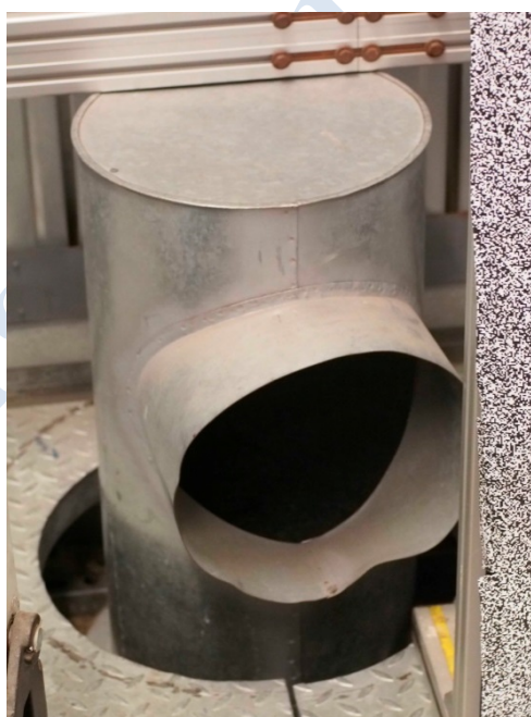
Figure 4-8. Pipe communicating the main volume of the facility and the underground room.
