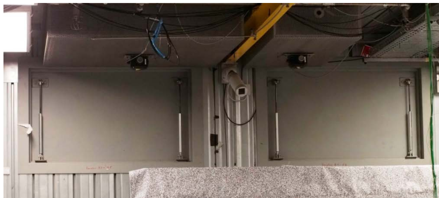
Figure 4-7. Flaps communicating the interior of the facility with the exterior environment.
